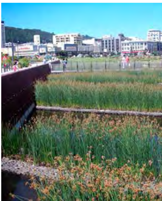
Figure 38. Innovative ways to provide green infrastructure within buildings will be investigated, the example above slows the water on its path to the stormwater system by using planting.
