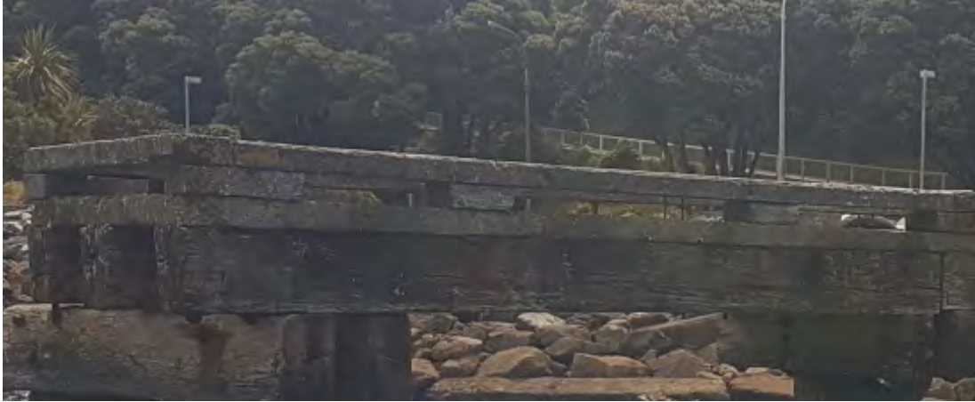
Figure 4-4. Cog Park Jetty – Representative View of All Joist
