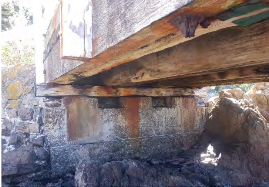
Figure 11-3. Karaka Bay Wharf – Concrete Abutment
