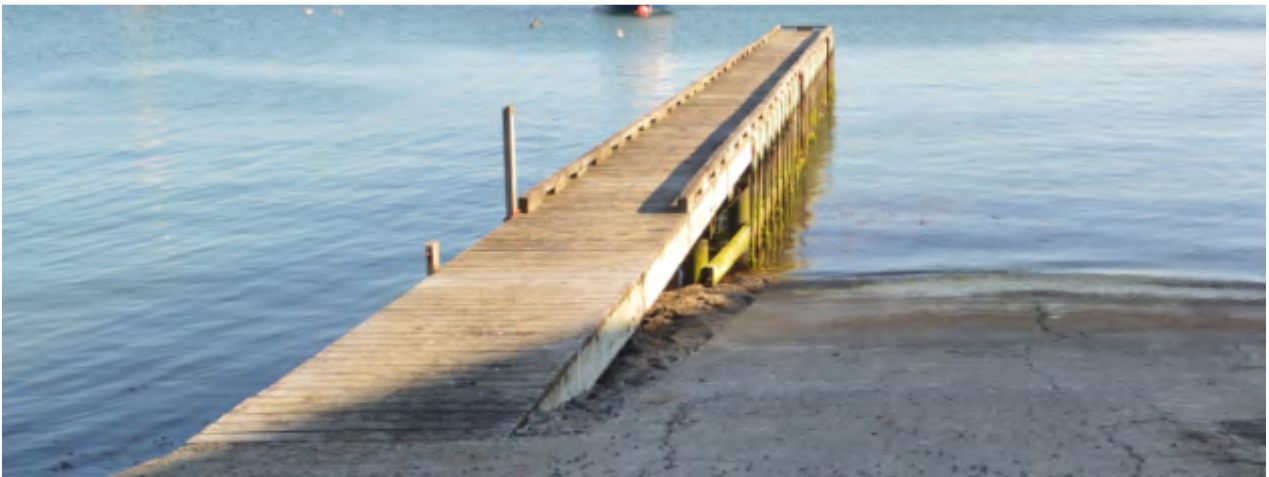
Figure 2-5. Greta point wharf – Decking
