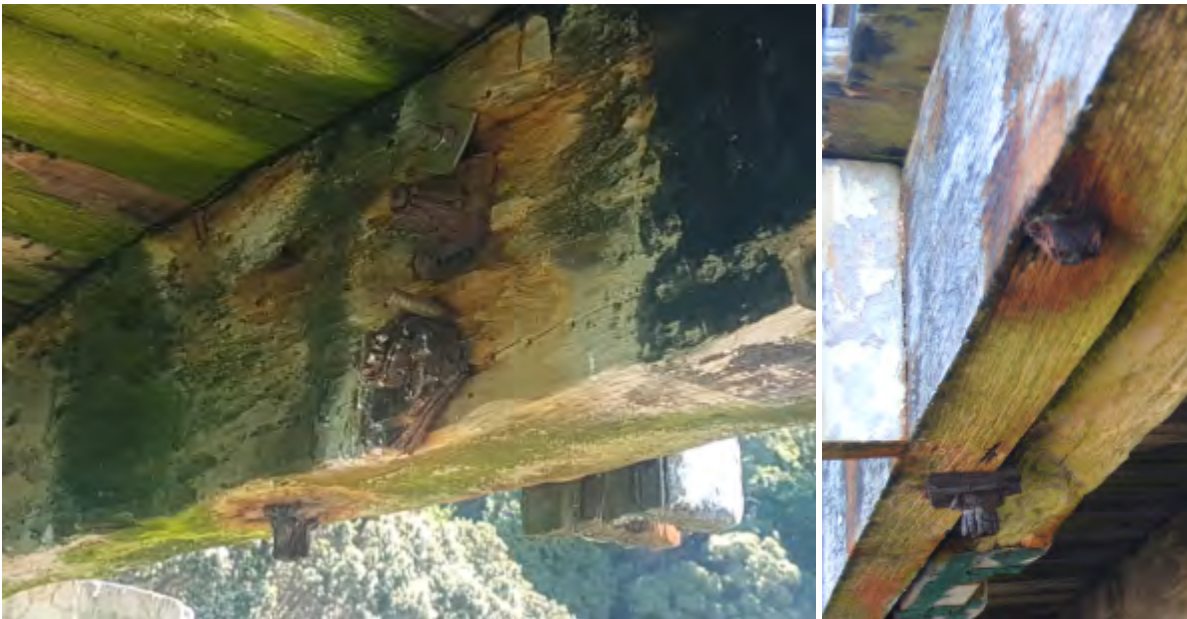
Figure 11-16. Karaka Bay Wharf – Bolted Connections of Original Joists and Decking Planks
