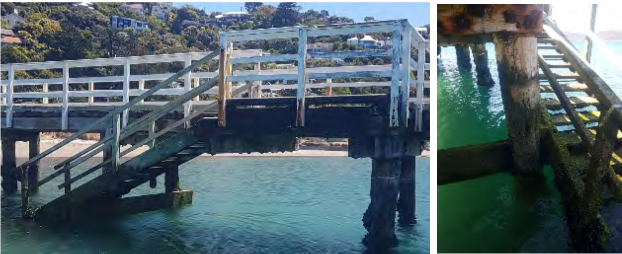
Figure 10-17. Seatoun Wharf - Stairs
