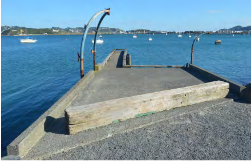
Figure 4-6. Cog Park Jetty - Top View on Concrete Deck
