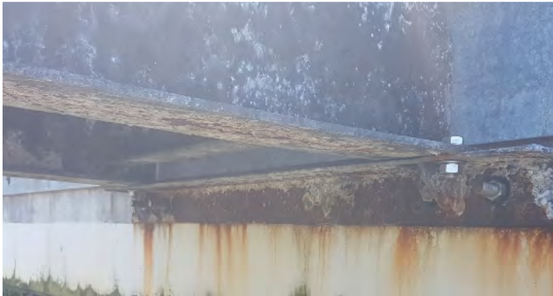
Figure 7-7. Evans Bay Yacht Club Travel Lift - Retrofitted Stainless Steel Connections
