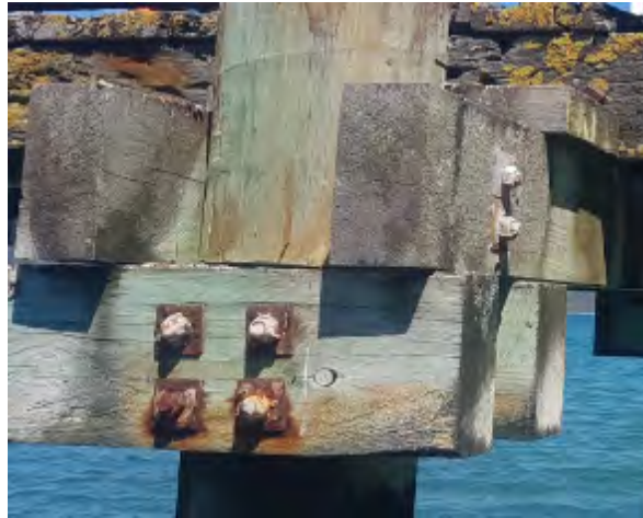
Figure 11-15. Karaka Bay Wharf – Bolted Connection of Underpinned Pier
