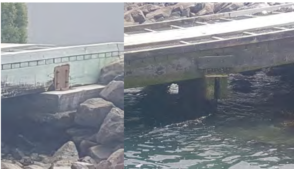
Figure 3-4. Cog Park Boat Ramp, Bolted Connections
