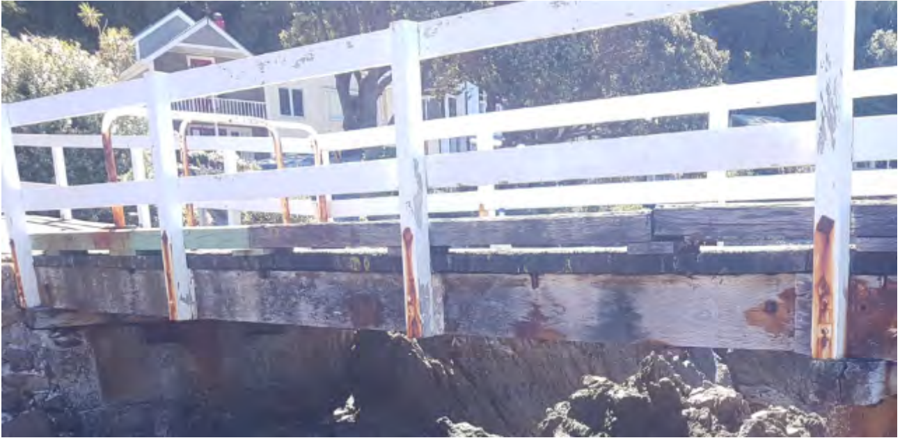
Figure 11-17. Karaka Bay Wharf - Handrail
