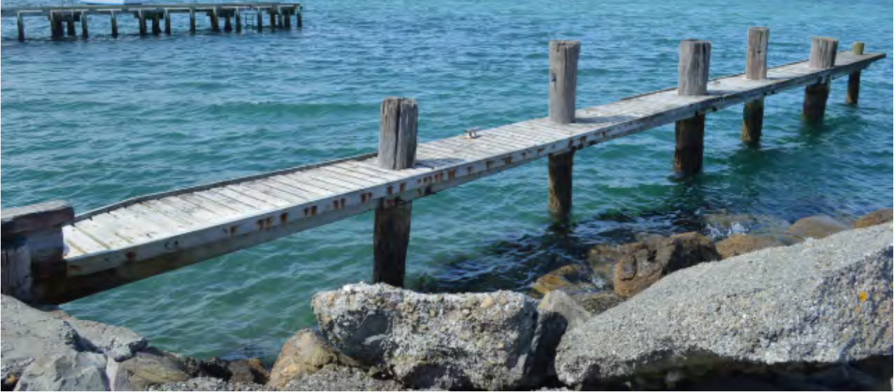
Figure 9-6. Evans Bay Boat Ramp South Jetty, decking
