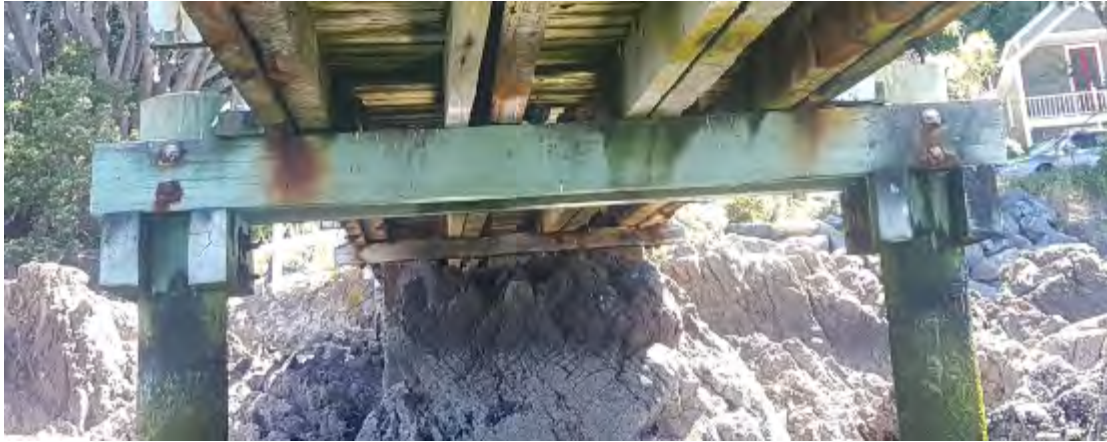
Figure 11-7. Karaka Bay Wharf – Bearers of Underpinned Piers
