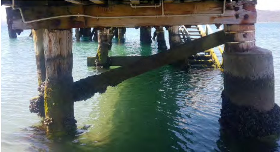
Figure 10-14. Seatoun Wharf – Bracing of Access Jetty
