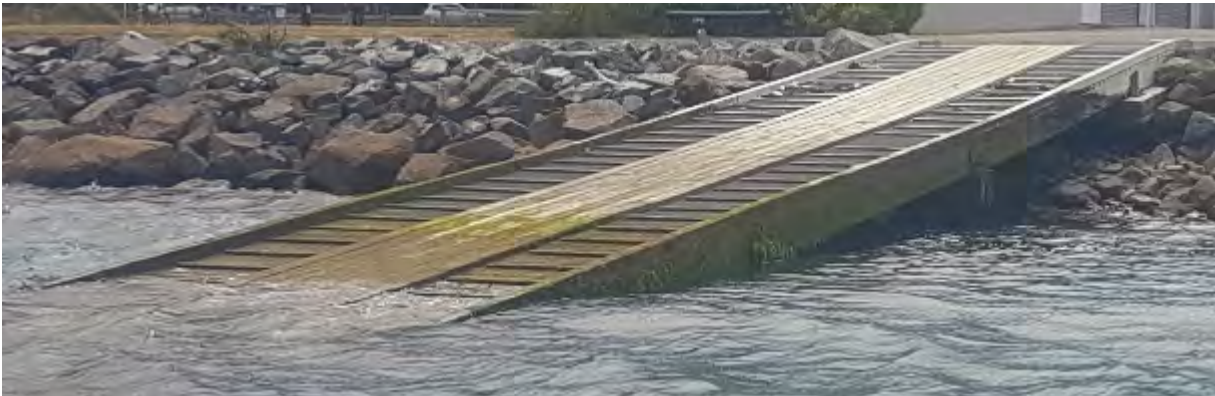
Figure 3-3. Cog Park Boat Ramp – Decking and Joist in Good Condition
