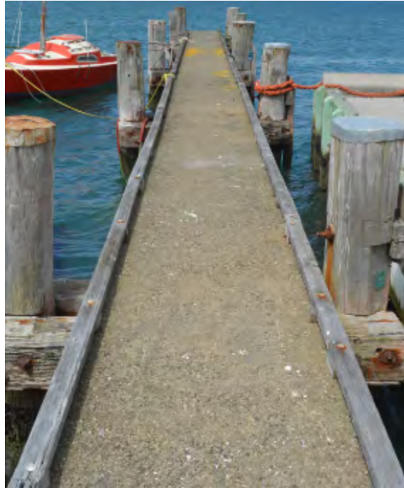
Figure 6-6. Evans Bay Yacht Club South Jetty - Top of Decking
