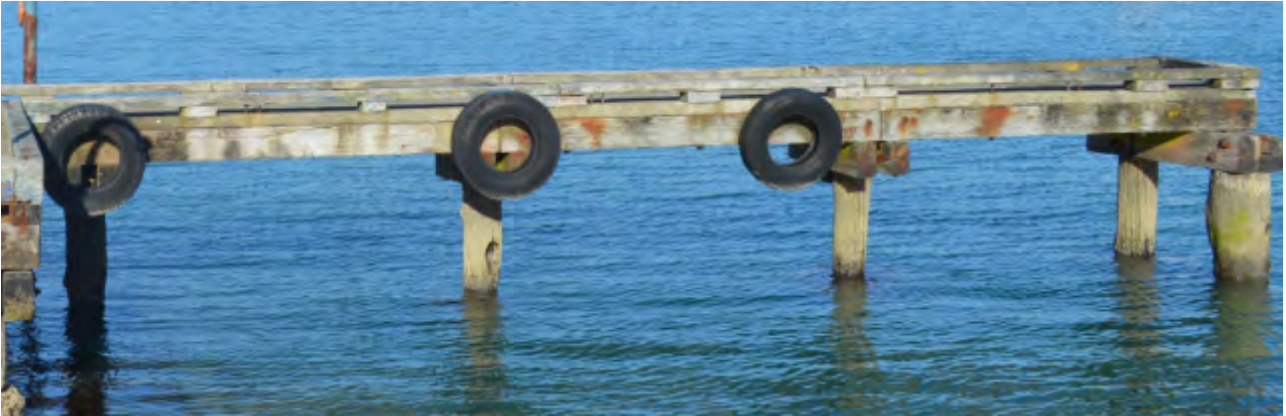
Figure 4-10. Cog Park Jetty – Tyre Fenders
