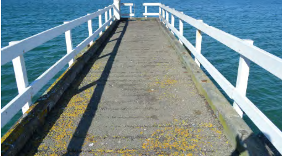
Figure 11-13. Karaka Bay Wharf – Top Side of Decking and Handrails
