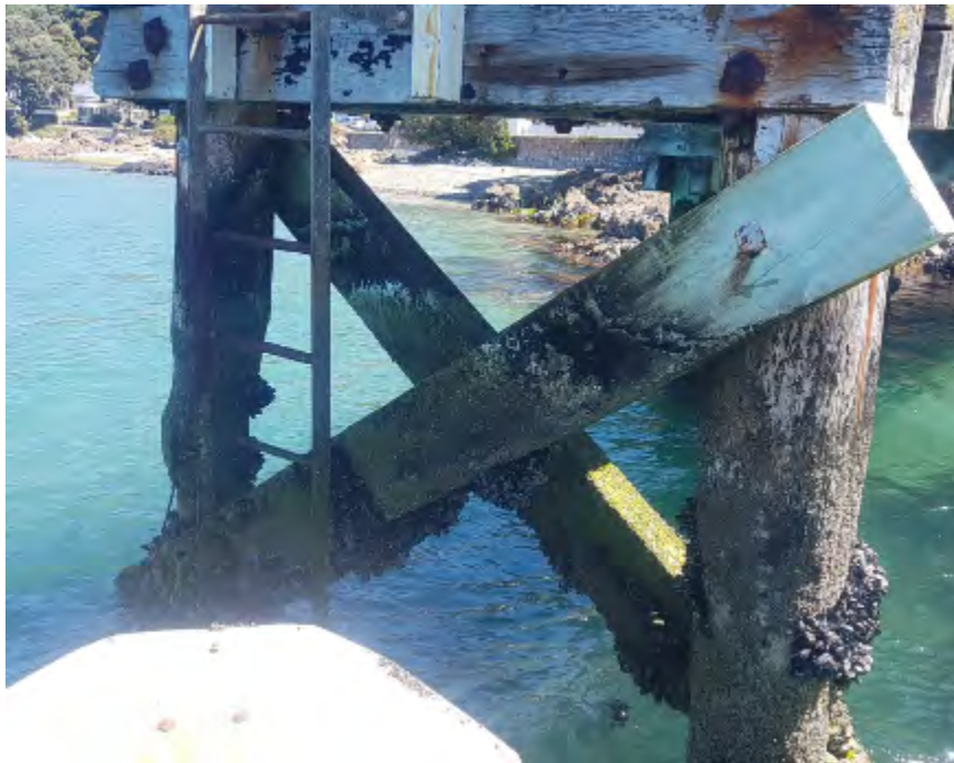
Figure 11-14. Karaka Bay Wharf – Bracing at End Piles
