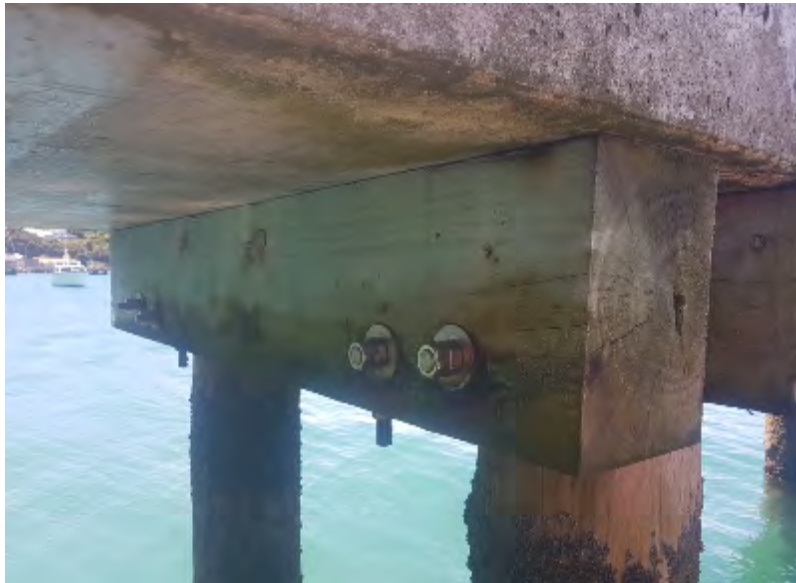
Figure 8-4. Evans Bay Boat Ramp North Jetty, Bearers and Connections
