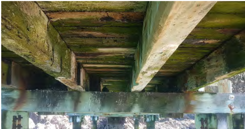
Figure 11-10. Karaka Bay Wharf – Joists in End Span
