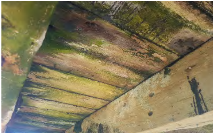
Figure 11-12. Karaka Bay Wharf – Underside of Decking
