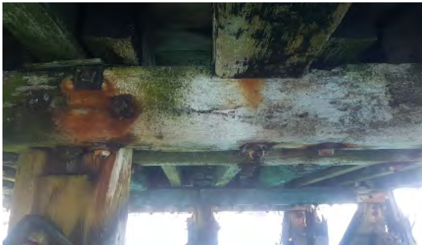
Figure 10-7. Seatoun Wharf - White Rot on Bearer, D2-E2
