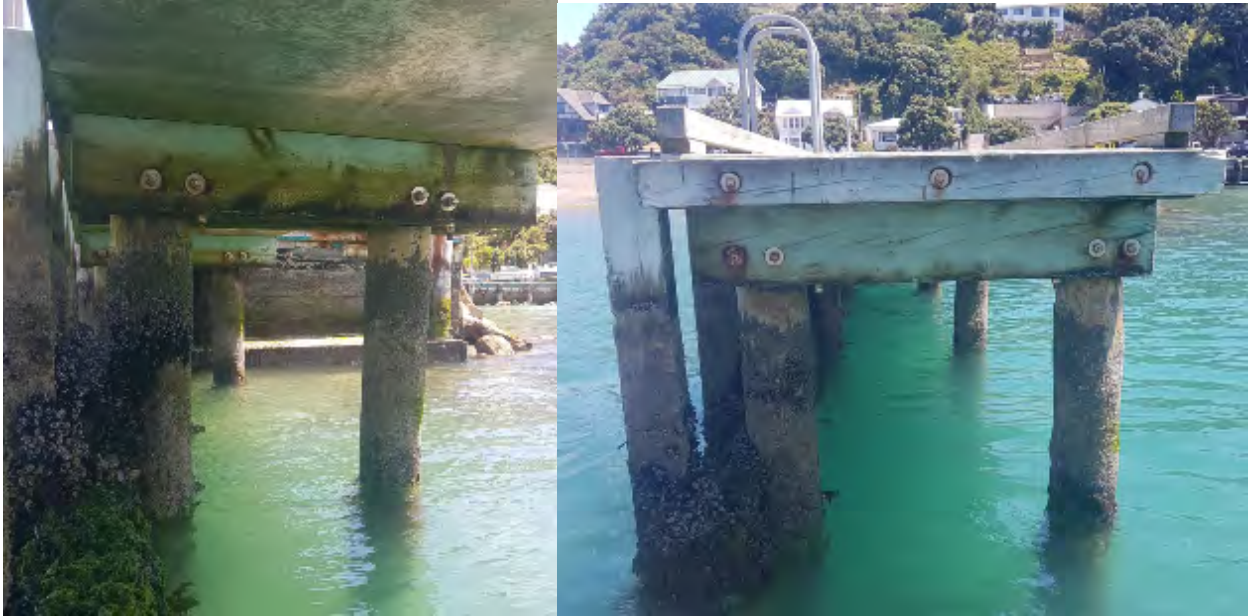
Figure 8-3. Evans Bay Boat Ramp North Jetty Piles
