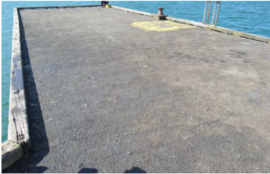
Figure 10-12. Seatoun Wharf – Mooring Platform Decking
