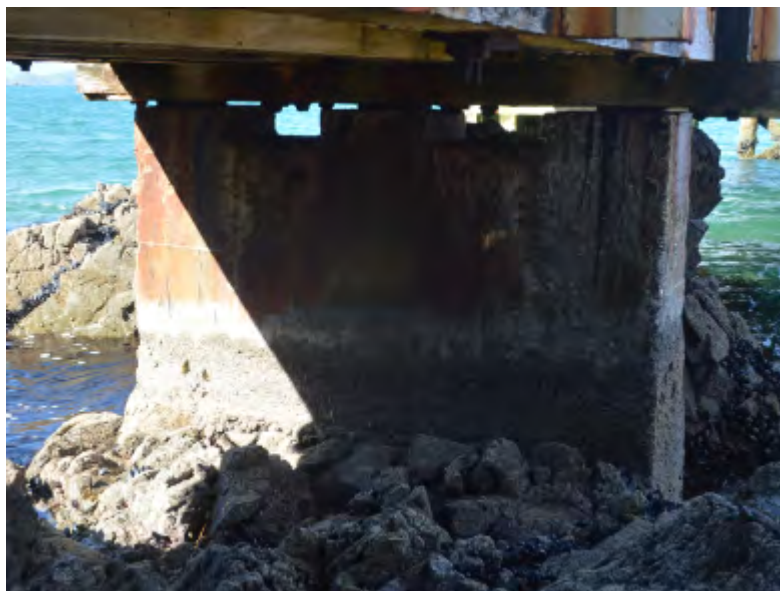
Figure 11-4. Karaka Bay Wharf – Concrete Pier
