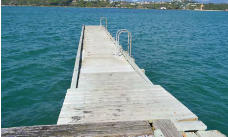
Figure 8-5. Evans Bay Boat Ramp North Jetty - Timber Decking
