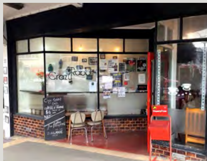
This attractive 1920s café at the corner of Waitoa Road and Moxham Avenue is a good example of a late Edwardian/interwar shop front.
