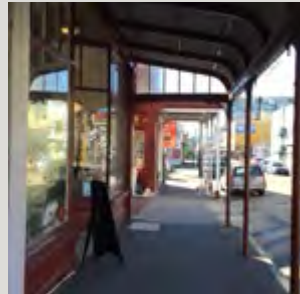
A bull-nosed verandah with clerestorey glazing
