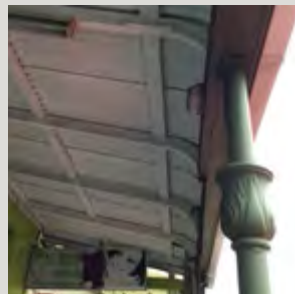
A bull-nosed verandah with cast iron posts
