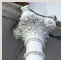
Cast iron verandah post
