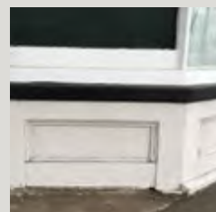
Timber panelled stall under the display windows
