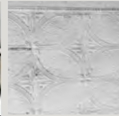
Pressed metal tiles verandah soffit
