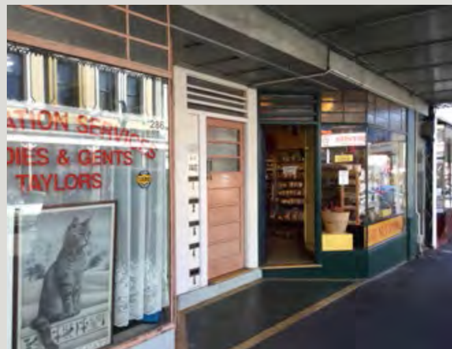
284-286 Cuba Street has two almost unaltered Art Deco/Modernist shop fronts.
