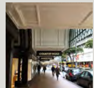
Pressed metal soffit
