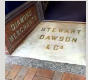
Signage on the entrance lobby and window stalls
